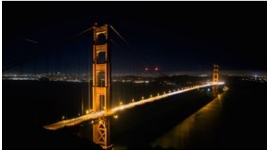
Time-lapse of San Francisco's Golden Gate Bridge.
